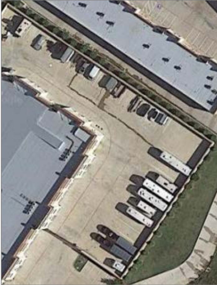
IMAGE 1: 2020 AERIAL IMAGE (GOOGLE)
